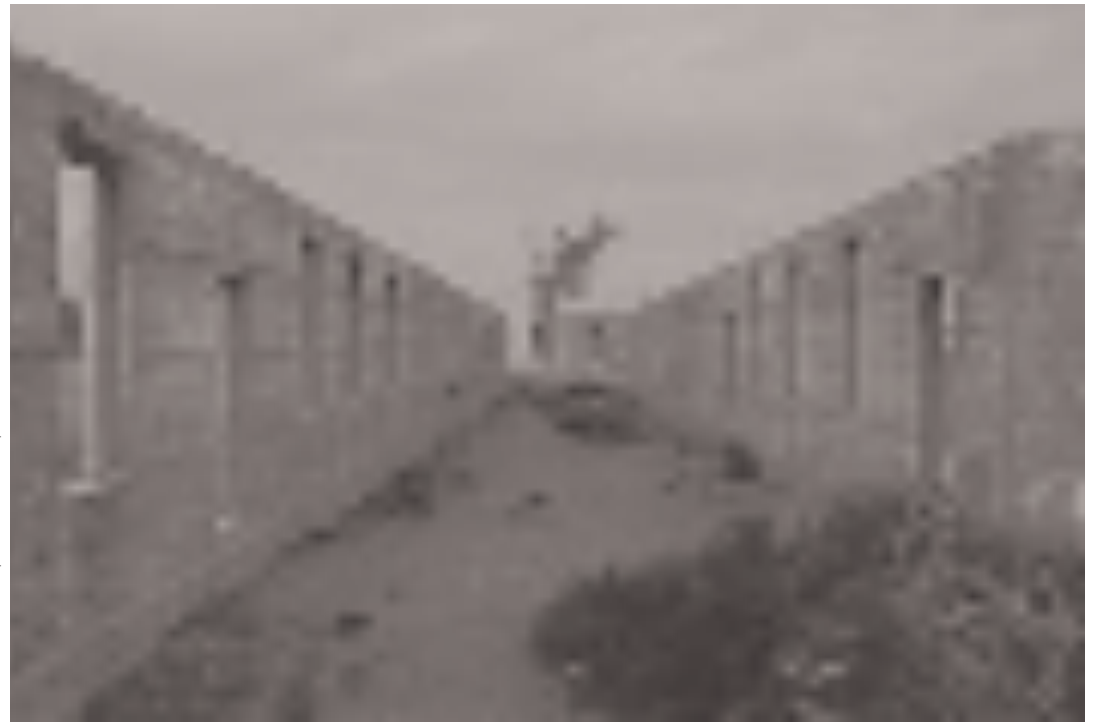
OLD HOSPITAL BUILDING, FORT D. A. RUSSELL, MARIETTA
